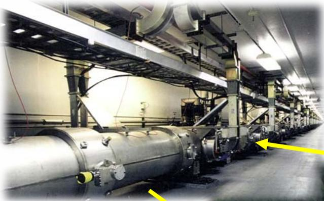
Cryomodules in the accelerator tunnel
